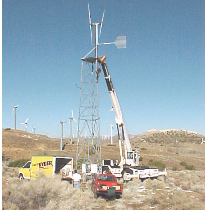
Figure 19. Contra Rotating Wind Turbine On a 50 ft Tower at Oak Creek Energy Systems Test Site
